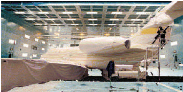
For large and small painting operations, 3M™ Clean-View Pads protect windows and light fixtures from overspray.
