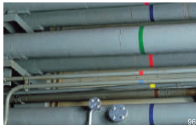
For color-coding pipes with 3M™ Vinyl Tapes, select from either nine vivid colors or transparent to let underlying color show through. Backing is colored throughout to help maintain ready visibility.
